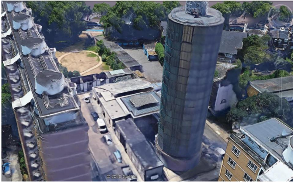
Figure 2 - Aerial view of PDHU Pump House and accumulator tower
